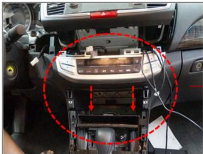
Pull out the Bolts
