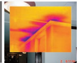
FUSION PIP Image of Water Leak: Hidden water leak from the ceiling
